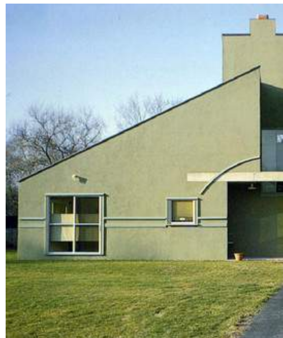
Robert Venturi, Vanna Venturi House, Philadelphia, 1959-1964
