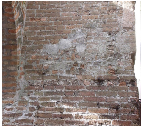
Fig. 12b- Venice: the remains of the previous medieval crenellated wall has been detected by stratigraphy (reconstruction by the author; graphic layout by the students Gianicola, Omelchenko, Zattarin, luav, a.a. 2014-15).
