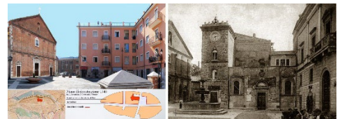
Fig. 17- Piazza Corradino compromised by the demolitions (1949 Reconstruction) (elaboration by authors, 2010).
