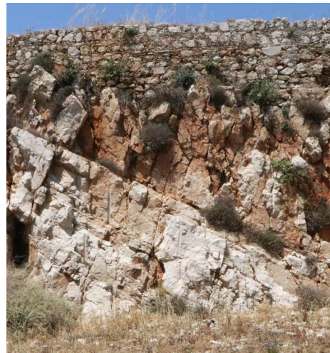
Fig. 9- The moat. Rock with drill holes for explosives
