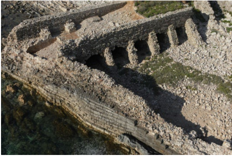
Fig. 7- The western bastion from the west. (P. Tokmakidis, 2024).
