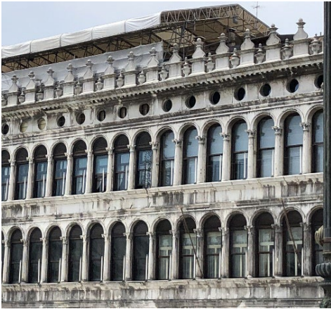
Fig. 5- Venice, Procuratie Vecchie: 16 th century articulated stone merlons in a representative public building (Angela Squassina, 2024).
