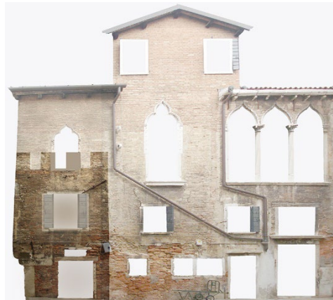
Fig. 12a- Venice: fragments of merlons and of a saw-tooth shaped frame are still detectable within the later façade of a gothic building (Cavallero & Nardi, 2014).
