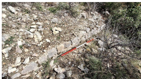
Fig. 7- Lines of the fortification wall (photo by Fortress of Culture, 2024).
