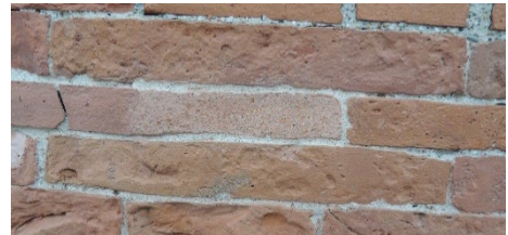
Fig. 18- Pink mortar restoring a brick, and decayed brick, Forte dei Marmi (photo by Silvia Rescic, 2024).
