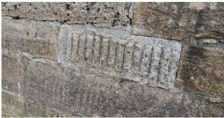
Fig. 16- Ribbon-like surface finish on pietra Panchina, Castagneto fort (photo by Fabio Fratini, 2024).
