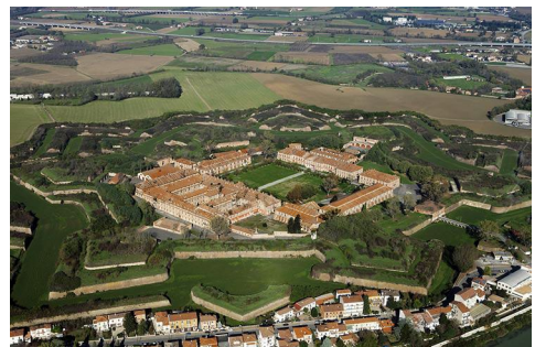
Fig. 5- Bastion general overview.
