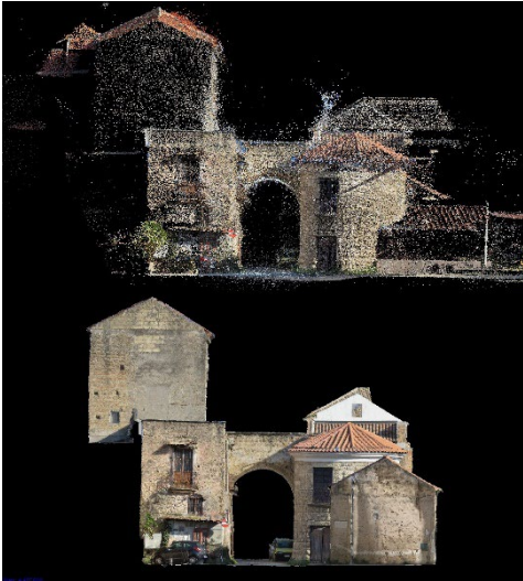
Fig. 3- Point cloud and texture models of the Porta San Giovanni and surrounding buildings. (graphic elaboration by authors, 2024).
