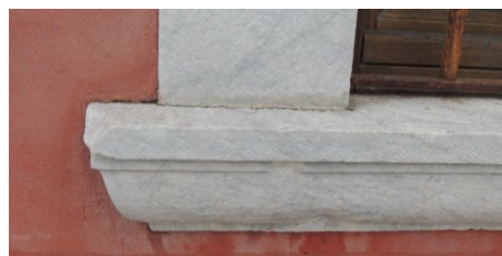
Fig. 11- Opening frame in white veined marble in Forte dei Marmi (photo by Silvia Rescic, 2024).
