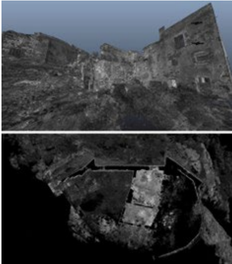
Fig. 8- Results from the TLS survey campaign, interiors of the tower (graphic elaboration by the authors, 2024).
