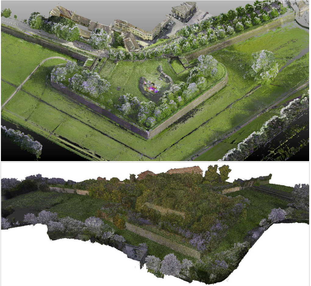
Fig. 11- Final integrated point cloud of Santa Croce (up) and Santa Cristina (bottom) bastions (graphic elaboration by author, 2024).
