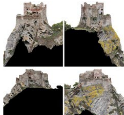
Fig. 14- Fronts of the main body of the tower produced by photogrammetry (graphic elaboration by the authors, 2024).
