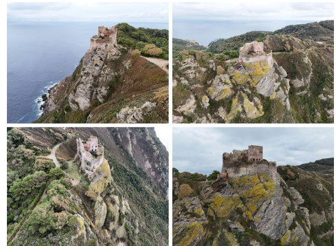
Fig. 10- Results from the UAV survey campaign, external fronts of the tower (photo by the authors, 2024).
