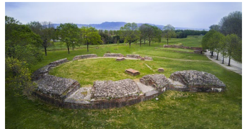
Fig. 3- Bastion general overview.
