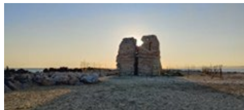
Fig. 3- View of the tower in its present conditions.
