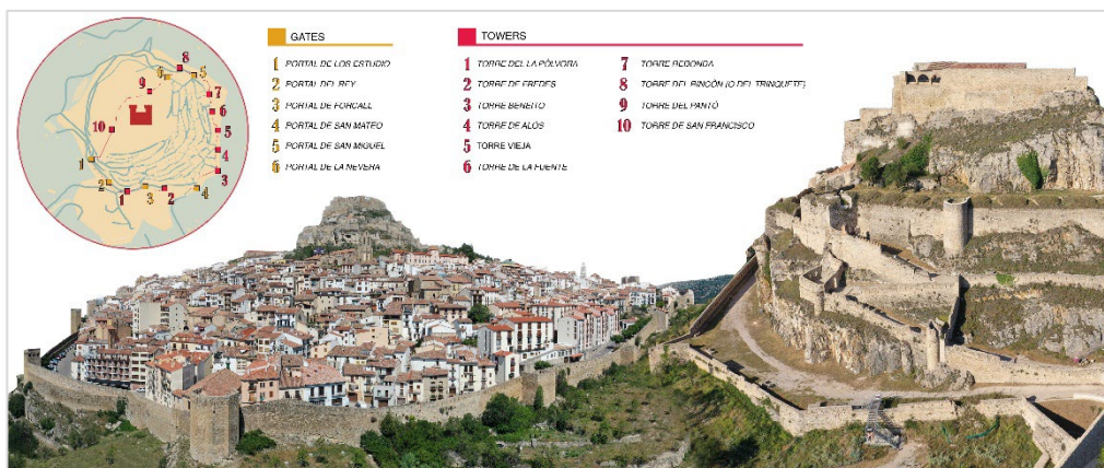
Fig. 1- The historical centre of Morella and its fortified monumental system. The core has 17 defensive elements including control towers and monumental portals, defending the central fortress Graphic elaboration by Francesca Picchio, Francesca Galasso, 2024.
