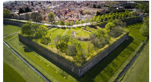
Fig. 2- Bastion general overview.
