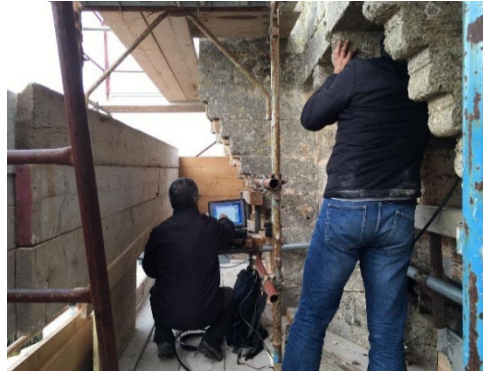
Fig. 2- Geophysical campaign: acquisition phase (photo by Author, 2019).
