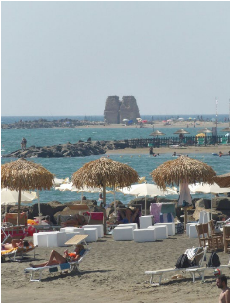
Fig. 4- View of the tower from the distance in its present state.
